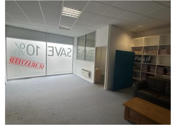
Partitioned office in rear corner
