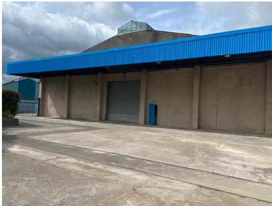
Rear loading door with canopy over.
