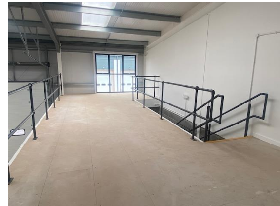
Mezzanine floor with first floor windows
