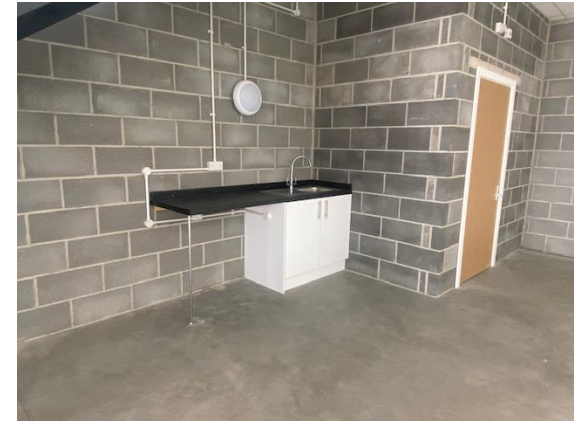
Tea station and toilet located on ground floor
