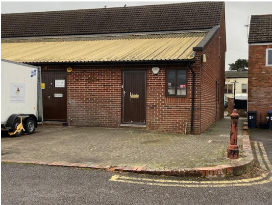
Parking spaces at rear of property
