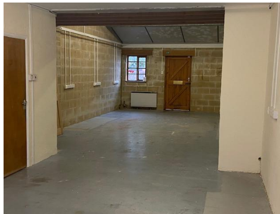
Looking toward the rear of the property.
