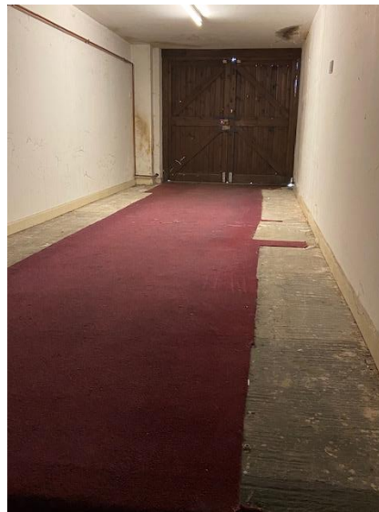
Ground floor rear storage and back doors.
