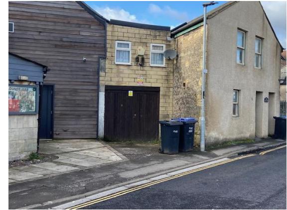
Rear doors and access
