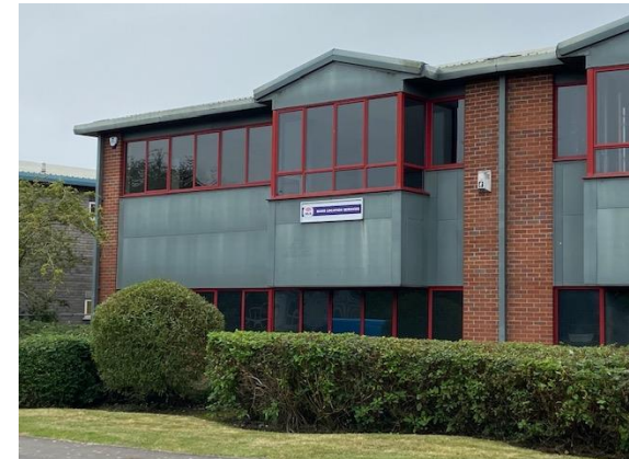
Redman Road frontage
