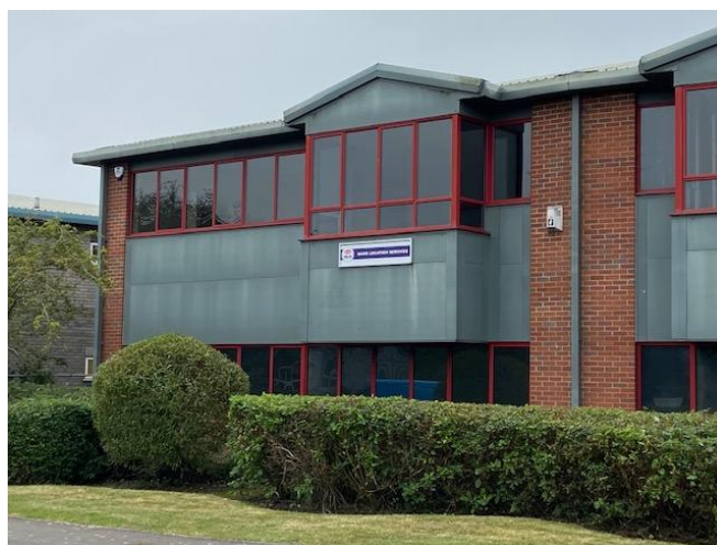
Redman Road frontage
